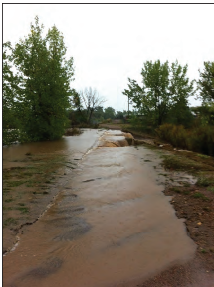
Top left: Damage to Bass Pond allows water to flow into Cottonwood Marsh.
