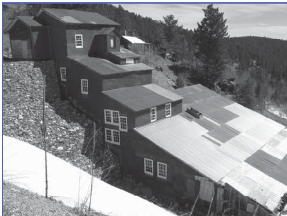
The Cardinal Mill building
