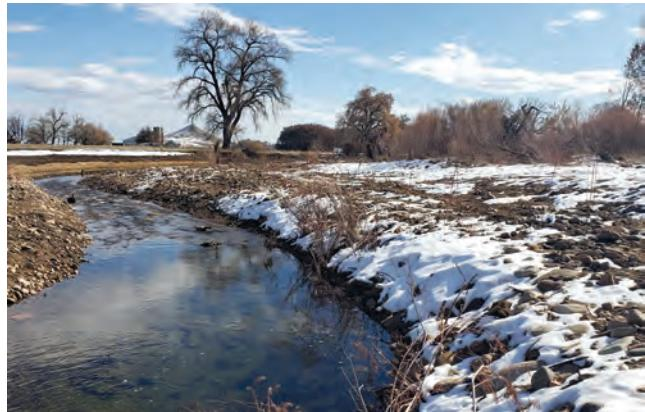
The department partnered with North State Environmental to reconstruct approximately 2,000 feet of stream at the Brewbaker Sorenson property. Work included creating a more sinuous channel alignment, bank stabilization using large wood and boulders, constructing riffles and pools, and floodplain grading. The project will improve the quality of the aquatic, riparian, and wetland habitat, restore stream function, and reduce future flood risk to the open space and neighboring properties.
