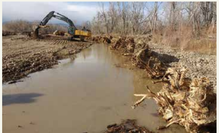
Active construction on St. Vrain Creek in 2018, installing large wood as bank protection and aquatic habitat
