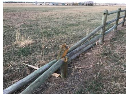
Photo 12. Damaged wooden rail fence near Ron Stewart Preserve (attributed to elk)
